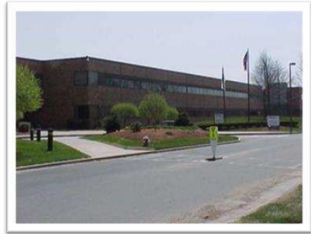
Photo: UMass System Office – Shrewsbury, MA
